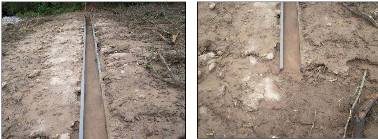
**Figure 4.** Sediment trap
