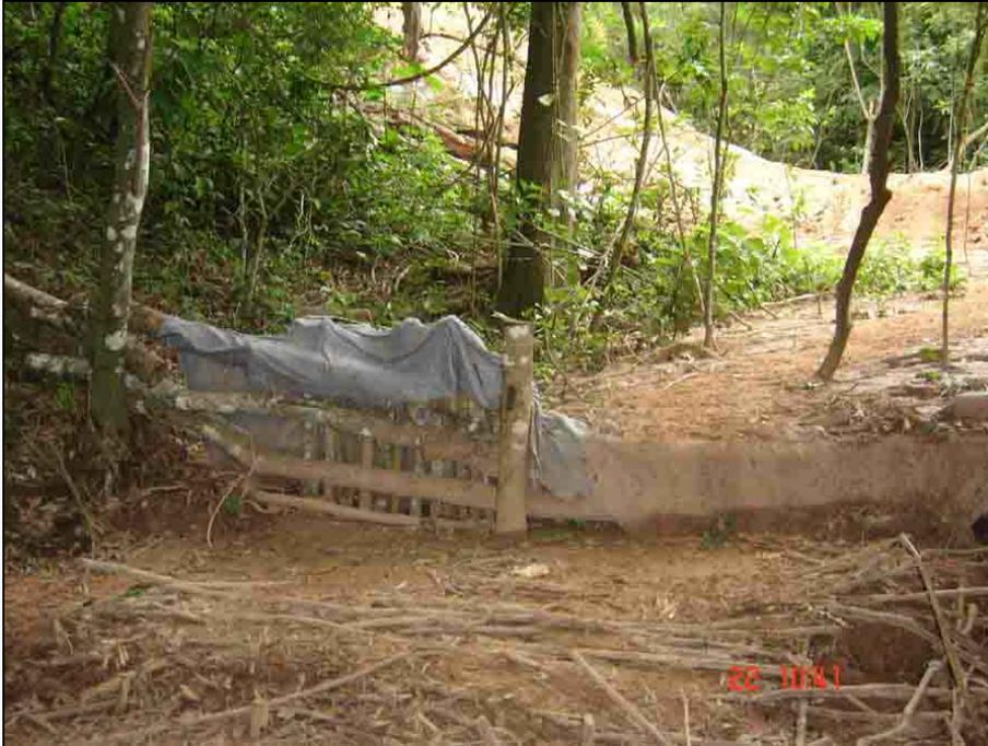
Figure 5. Silt fence
