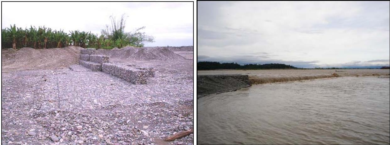
**Figure 1.4.** View of one groin at dry conditions and during the passage of a flood wave
